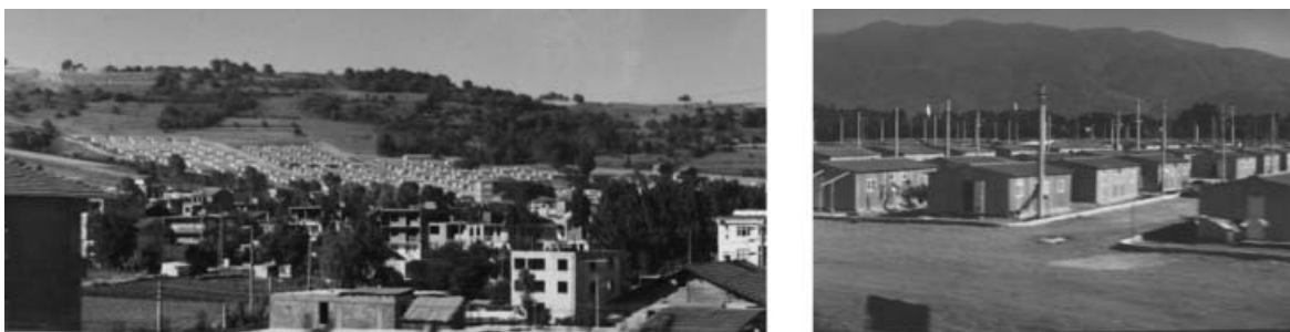
Figure 4 Views of the temporary housing settlement built in the outskirts of the cities of Adapazari and Izmit
