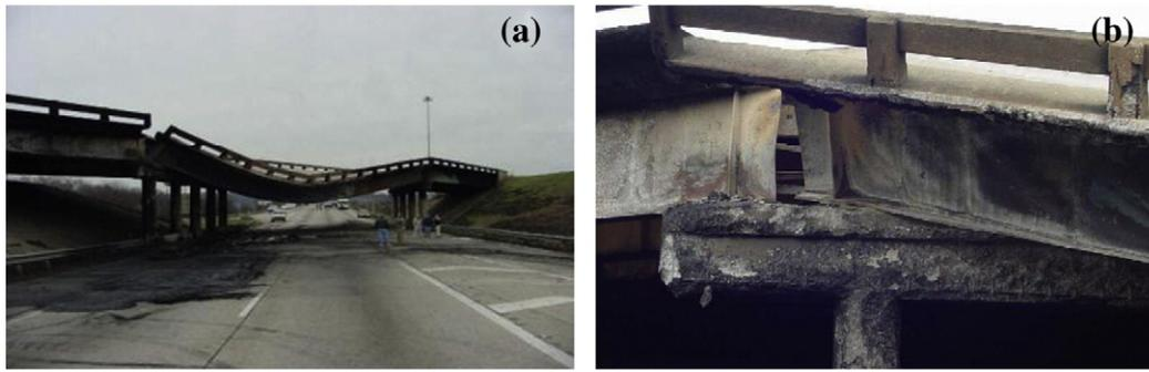
Fig. 1. I-20/I-59/I-65 interchange in Birmingham, AL after a fire: (a) severe deflections in the steel girders, and (b) web shear buckling observed near the bent cap. Photos courtesy of the Alabama DOT.
