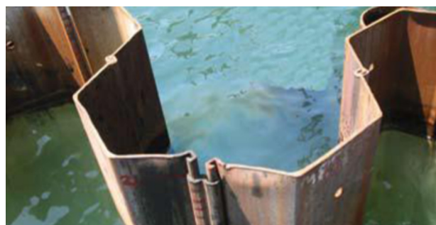
Fig. 3. Jagged sheet pile wall.
