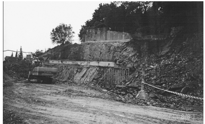
Fig. 7. View of the collapsed wall. The intact part of the wall with the cap beam can be seen on the left, and the failed part on the right.
