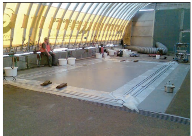
Fig. 8: Application of adhesive using vacuum infusion
