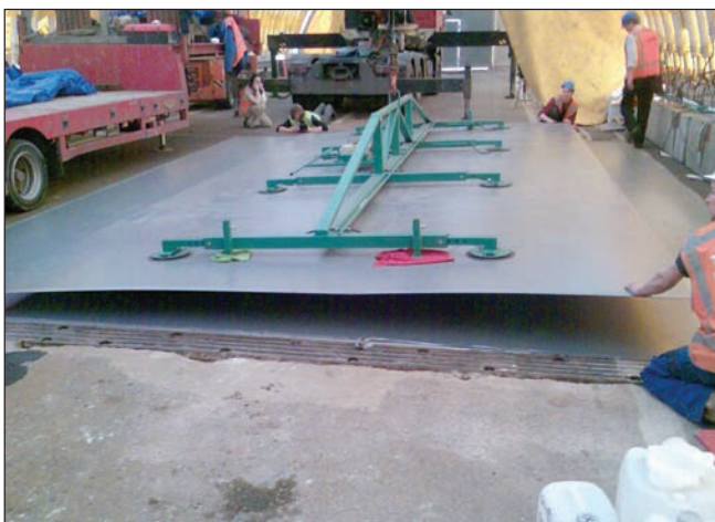
Fig. 7: Application of primed additional steel plate
