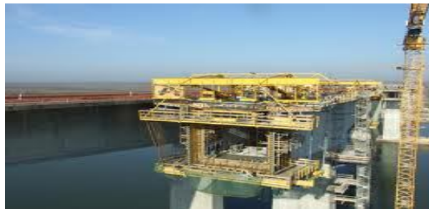
Figure 6. The structure of in-situbalanced cantilever
