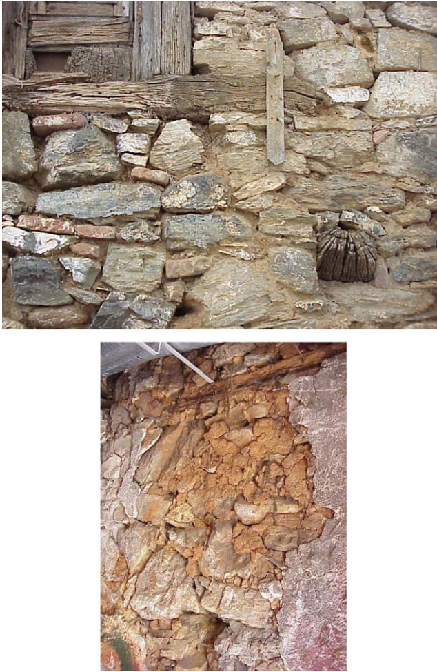
Fig. 5. Typical examples of masonry for external walls.
