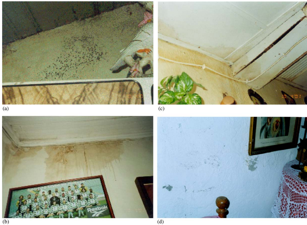
Fig. 13. Examples of the damages observed inside the houses: (a) biologic activity, (b) stains due to humidity, (c) timber and roof deterioration, (d) detachment of rendering and painting and efflorescence with high presence of salts.
