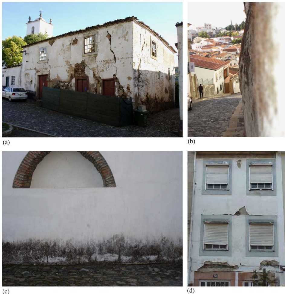
Fig. 7. Example of damage: (a) collapsed structures, (b) bulging walls, (c) stains in walls at soil level, (d) detachment of rendering and painting, (e) cracks, (f) mould, fungus and vegetation, (g) roof deterioration, (h) timber deterioration in openings frames or balconies.
