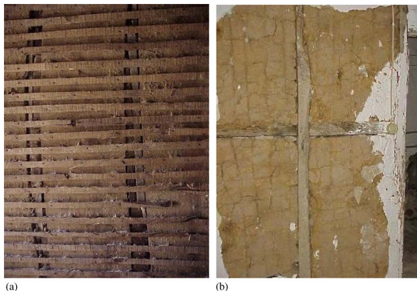
Fig. 6. Example of internal walls: (a) wooden lath walls and (b) “fachwerk” type.
