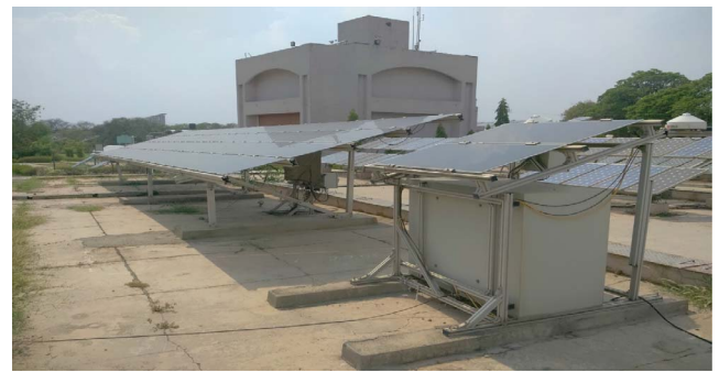
Fig. 3. 3.2 KW PV system with reference PV module and Pyranometer.
