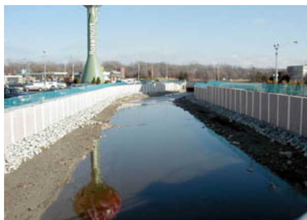
Floodwalls along Willow Creek in Rosemont, Illinois. Source: Kevin D. Richards, U.S. Geological Survey.
