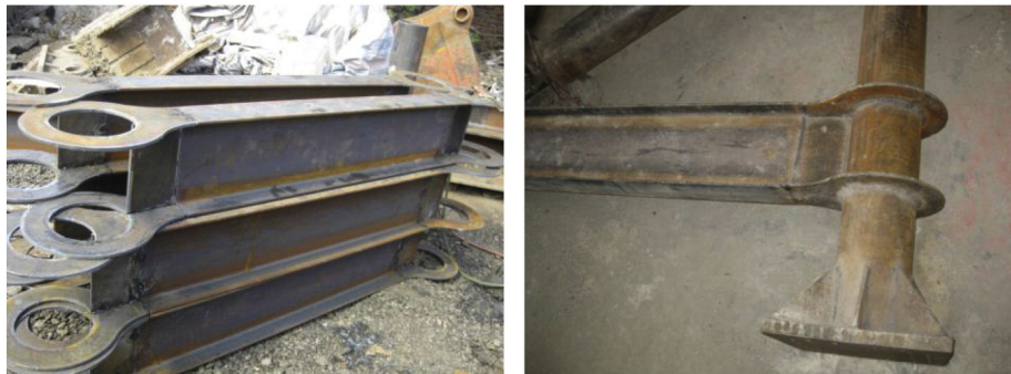
Fig. 5. Beam-column connection details.
