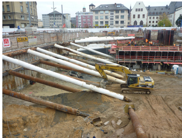
Fig. 4. Retaining structure in the north of the excavation
