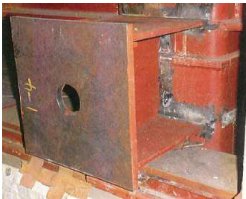
Figure 18. Bracket after welding work
