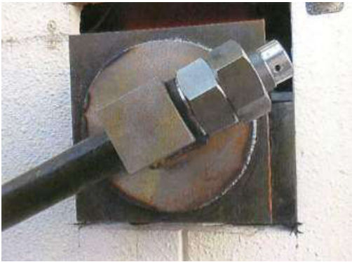
Figure 26. Completion of tightening double steel sleeve nuts
