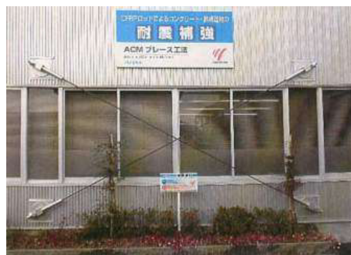
Figure 30. Completion of ACM brace installation
