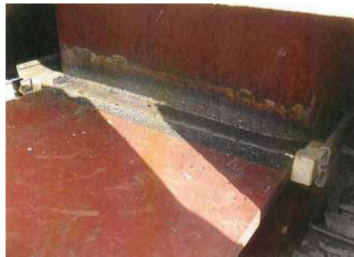
Figure 17. Completion of welding work of steel bracket
