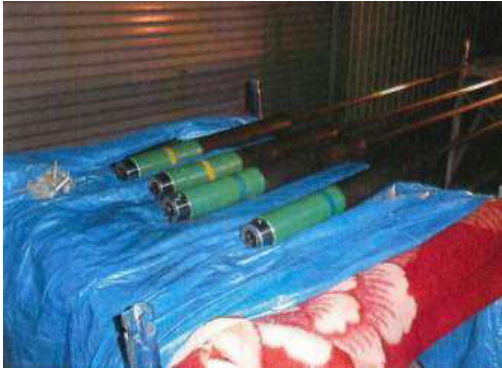
Figure 22. Steel sleeves before Epoxy resin Injection
