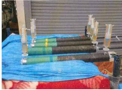
Figure 23. Epoxy resin injection work into steel sleeves
