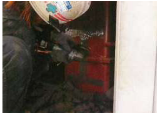
Figure 15. Polishing work on steel column before welding work of steel bracket
