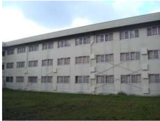
Figure 9. Completion of ACM braces
