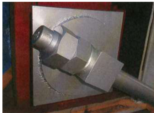
Figure 29. Steel sleeve and bracket after finishing painting work
