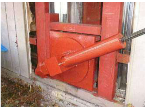
Figure 28. Steel sleeve and bracket after anti-rust painting
