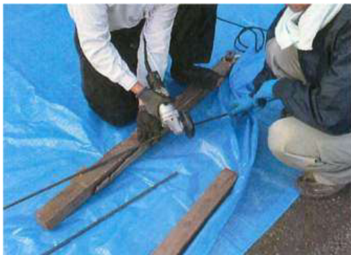
Figure 20. CFRP rod cutting work
