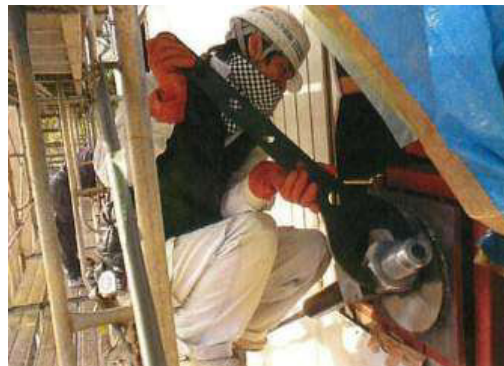
Figure 25. Tightening work of steel-nut with a screwdriver
