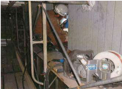
Figure 16. Welding work of steel bracket and a welder
