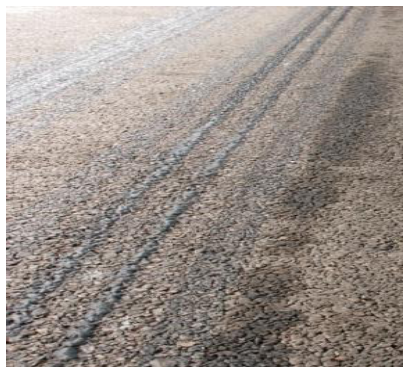
Figure 6: Rutted section
