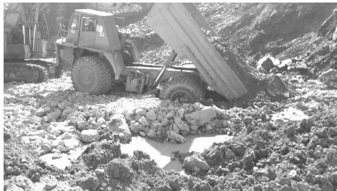
Fig. 10. Truck stuck in schist, inability to transfer load of the schist working space.
